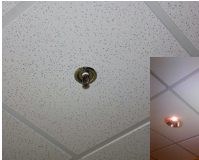
Incorrect sprinkler head positioning (right) compared to correct sprinkler positioning (left).
