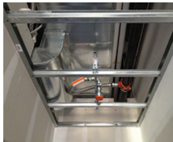
Flexible drop installed in crowded ceiling space.
